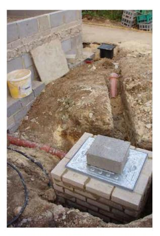
Seeing the pipe on the bed allows warranty inspectors to ensure that it's straight and the bed is correct. This is important because it reduces the possibility of bellies (where the pipe drops between joints or over an extended length). This is normally caused by poor preparation of the bed under the conduit, and if not corrected can cause constant blockages.
